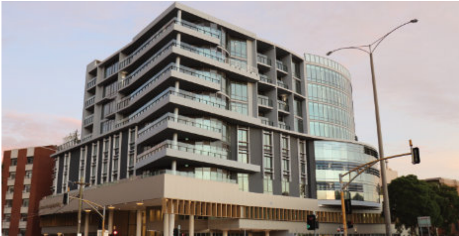
The Hannah & Daryl Cohen Family Building gets finishing touches.
